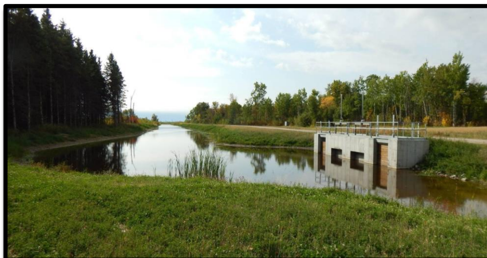
Pool 3 Outlet Structure
